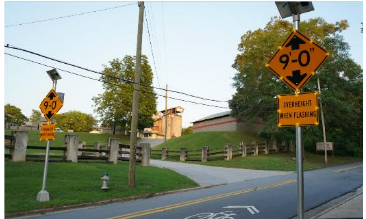
FIGURE 9. EXAMPLE OF A VERTICAL CLEARANCE WARNING SYSTEM
